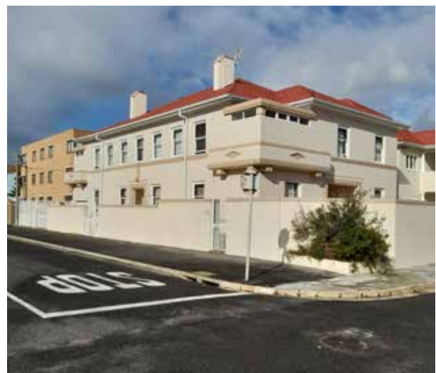
Watson Road renovation.
